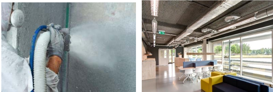
Figure 6: Cellulose insulation in sprayed application (left side the installation process – right side the installed product)
