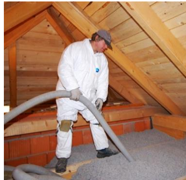
Figure 3: Cellulose insulation in open attics
